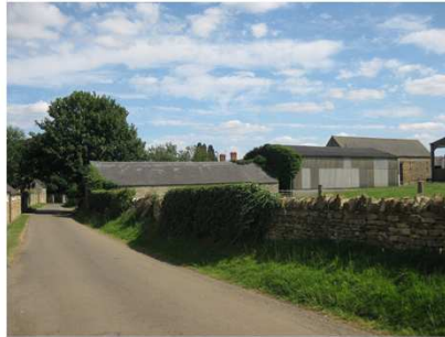
The stone boundary wall and verge on the south side of Back Lane, included within the Conservation Area.
